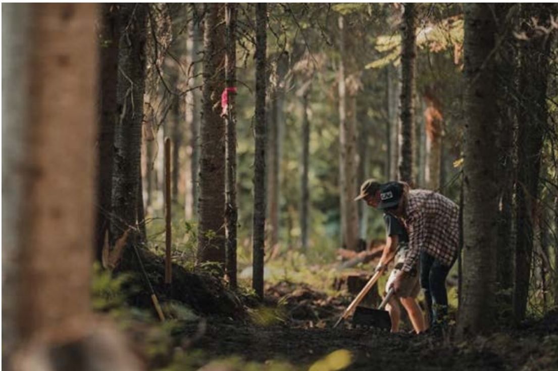
Work on Mt. Morrisey Destination Trail
