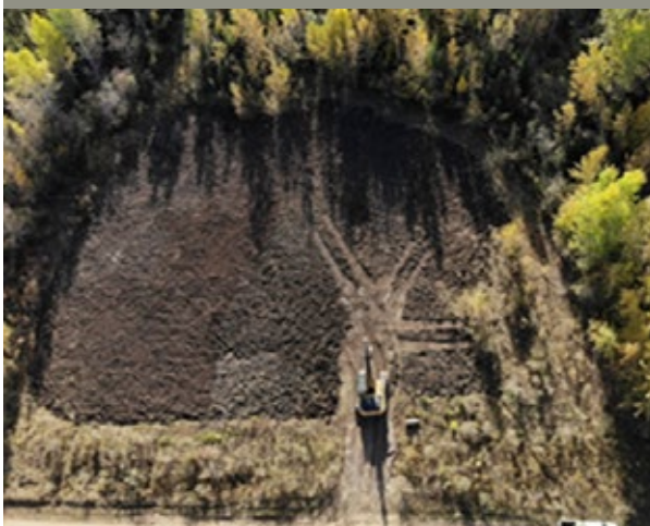
Exhibit 16: Excavating contaminated soil as part of site remediation
