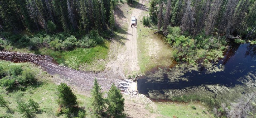
Low-consequence dam in northern B.C.
