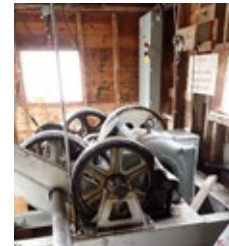
Right: Elko Dam in the Kootenay Region—dam spillway gate opening system (significant-consequence dam).
